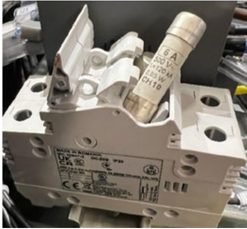
4 - CARTRIDGE FUSES 2X (10X38)MM 6A
